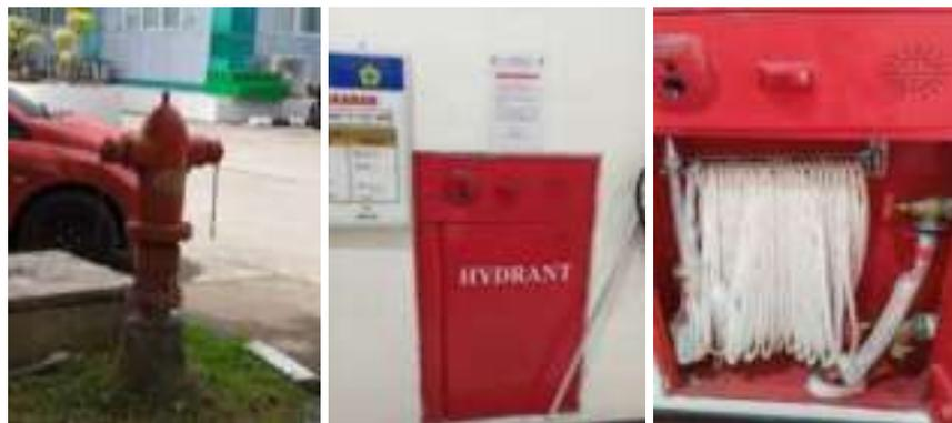
**Gambar 11. Kotak Hydrant Dan Pilar Hydrant**
